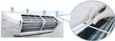
5. Slightly open the lower part of the front panel then pull the upper part of the front panel toward you to remove it as shown on figure.
